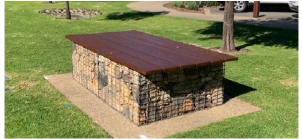
Gabion walls with timber slatted top
